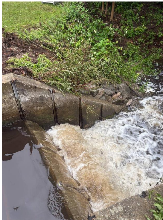
Photo 7 – Left downstream embankment during drawdown. (7/1/2026– Provided by the Village)
