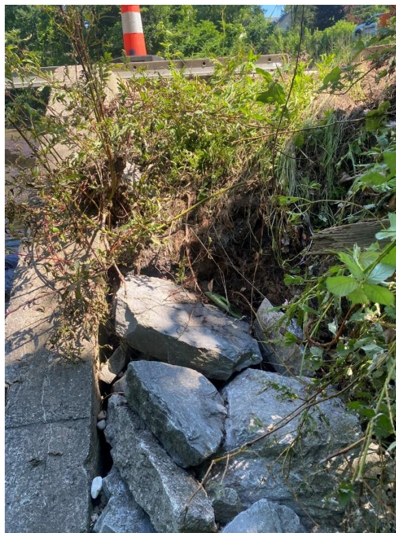
Photo 17 – Left downstream embankment looking toward the reservoir. (7/7/2026)
