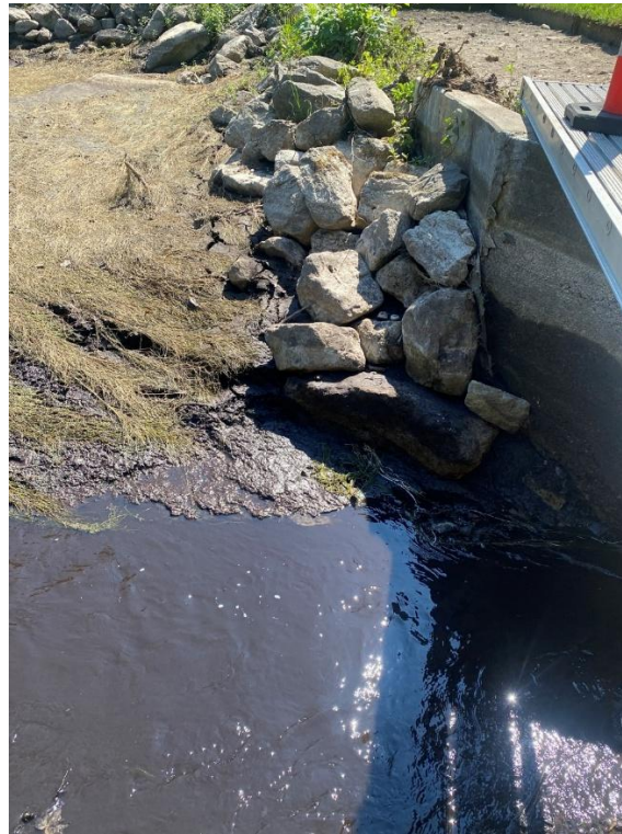
Photo 11 – Left upstream embankment looking eastward after dewatering. (7/7/2026)
