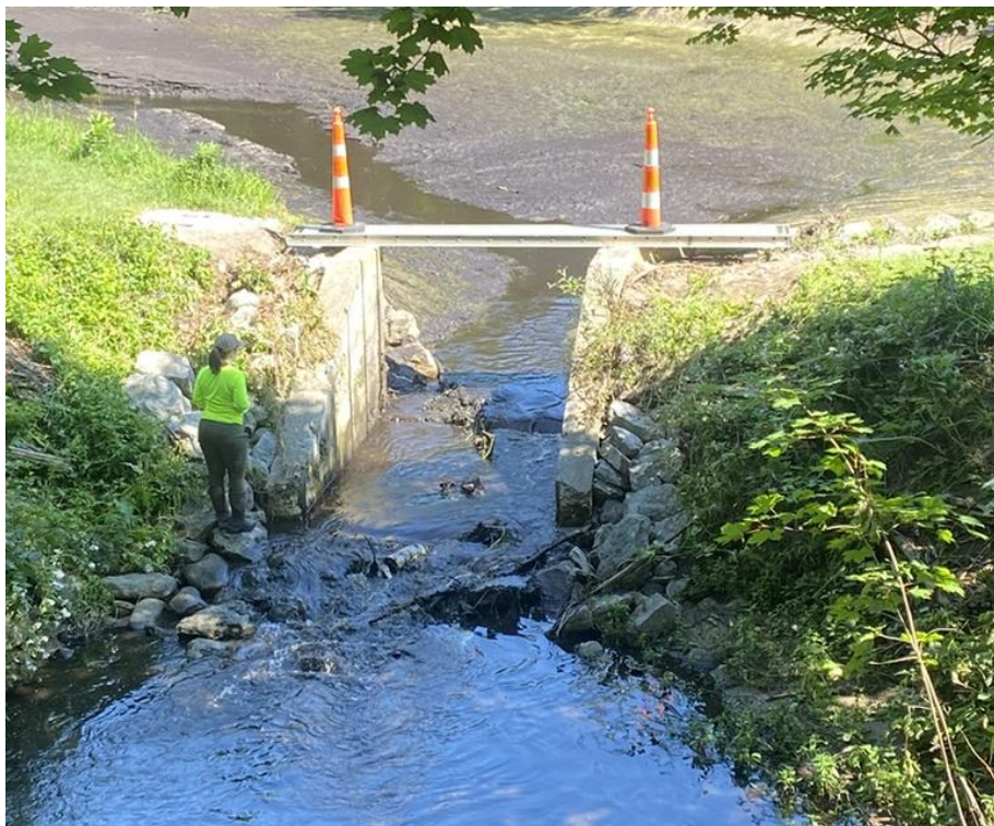
Photo 8 – Looking upstream at the concrete spillway after the stop logs were pulled. (7/7/2026)
