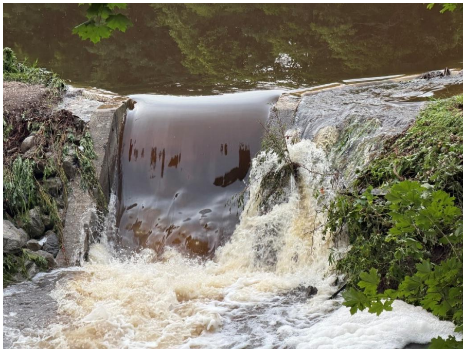
Photo 4 – Looking upstream towards the concrete structure before the stop logs were pulled. (6/30/2026 – Provided by the Village)
