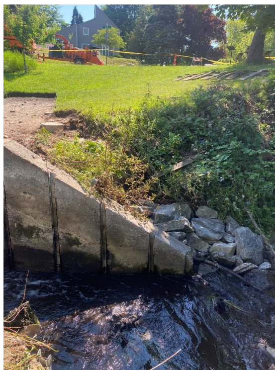
Photo 16 – Left downstream embankment and left training wall. (7/7/2026)
