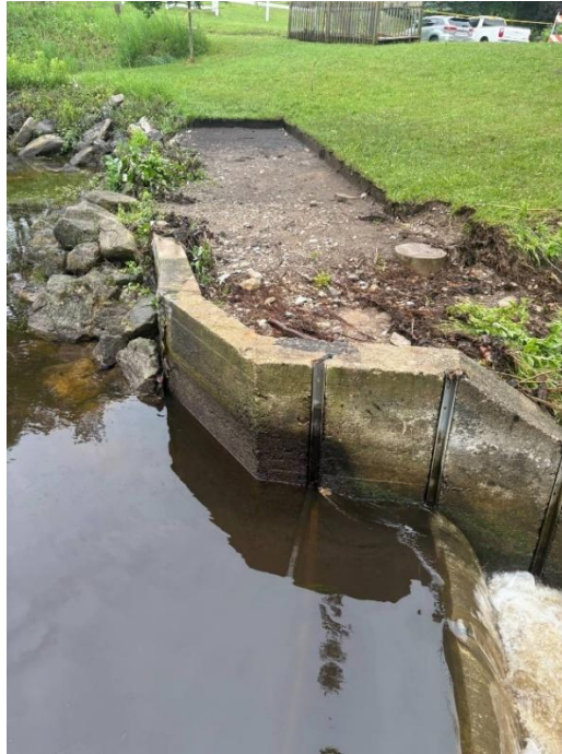
Photo 5 – Left embankment looking from the right embankment during dewatering of impoundment. (7/1/2026– Provided by the Village)
