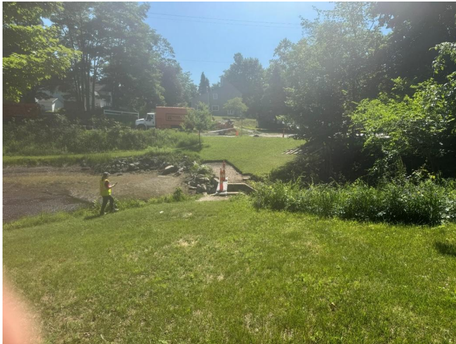
Photo 9 – Right embankment looking eastward from the right abutment. (7/7/2026)
