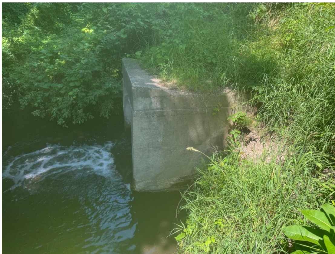
Photo 20 – Downstream end of 3 rd Street culvert looking from the left. (7/7/2026)
