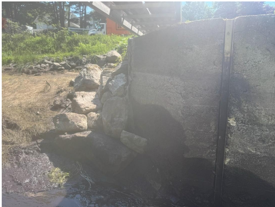
Photo 12 – Left upstream embankment after dewatering looking eastward. (7/7/2026)
