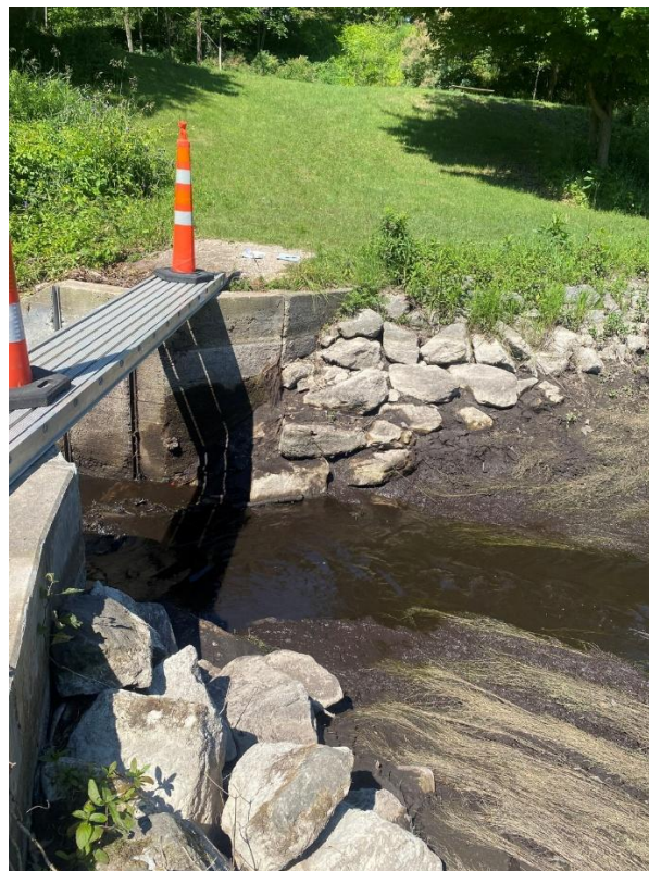
Photo 10 – Right upstream embankment looking from the left embankment. (7/7/2026)
